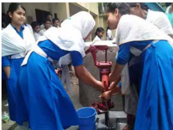
Students taking water from CWB ring well at Terail High School
