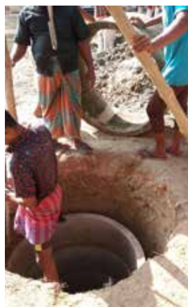
Installing the rings
