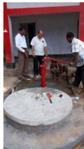
Installing the pump & finishing the well
